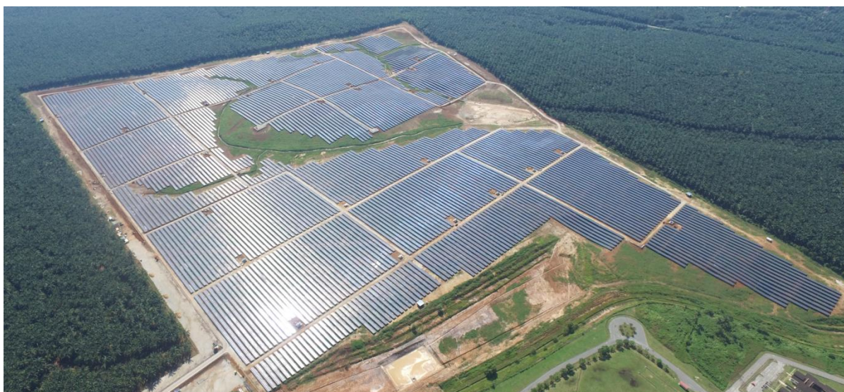
Picture Caption: Aerial view of the Tianjin Electric Power Construction – Kuala Ketil 50MW Solar Power Plant Project, Kedah, Malaysia
