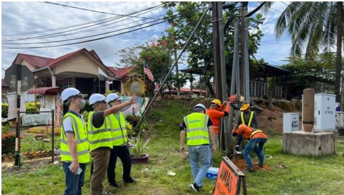
Picture Caption: Construction site of wireless and fiber networks in rural Malaysia, enhancing local connectivity capacity
