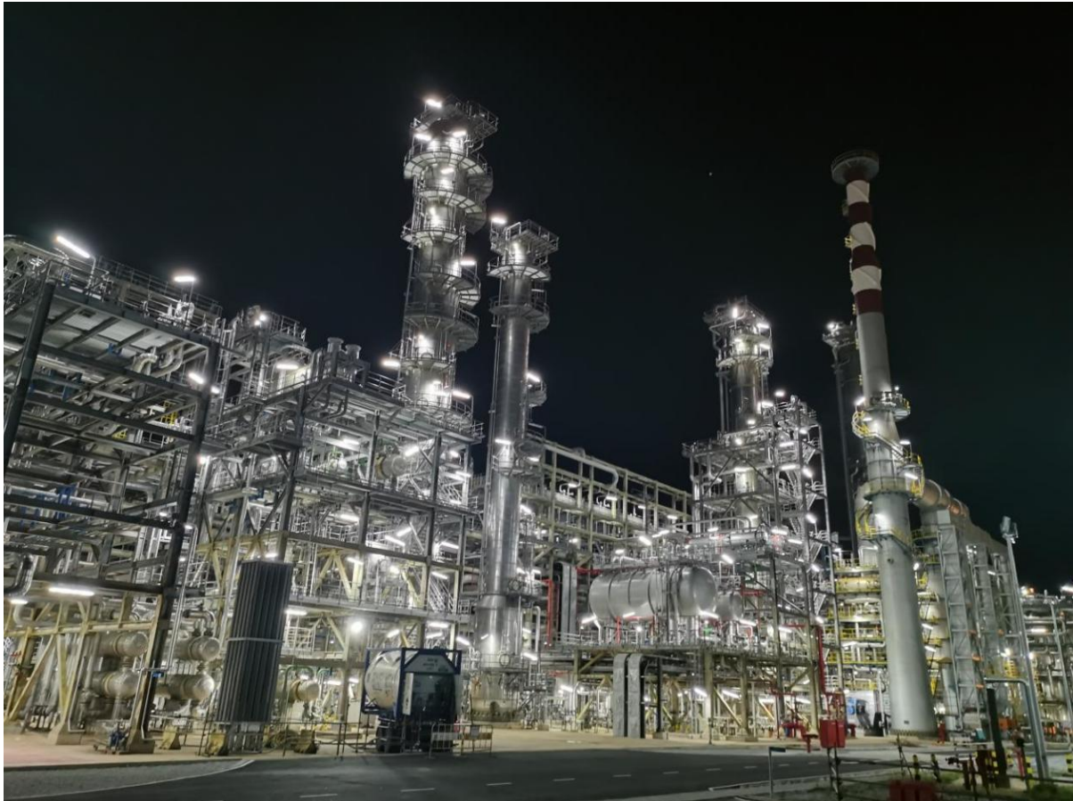
Picture Caption: Hengyuan Refinery
